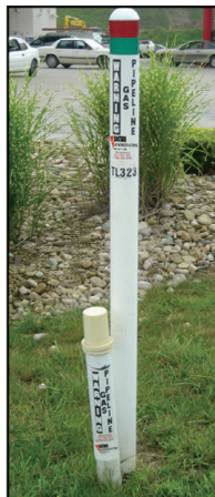
2. Linemarker and cathodic protection test station
